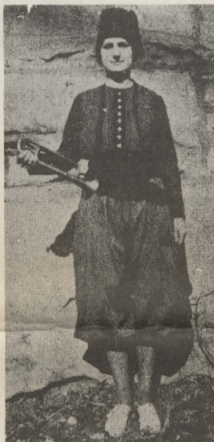
Picture taken of myself against the culvert wall with my bugle.
